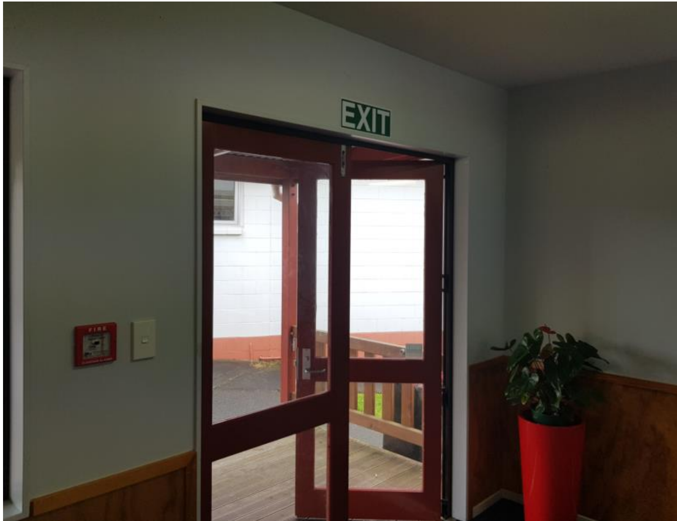
Fire Exit/Call Point at the Parish Hall Main Entrance
